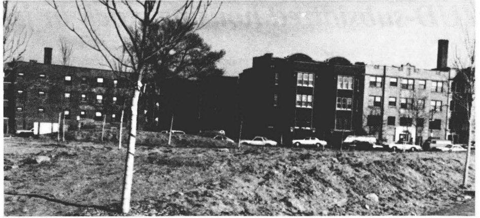
The HSC property owners program works with buildings such as these.
