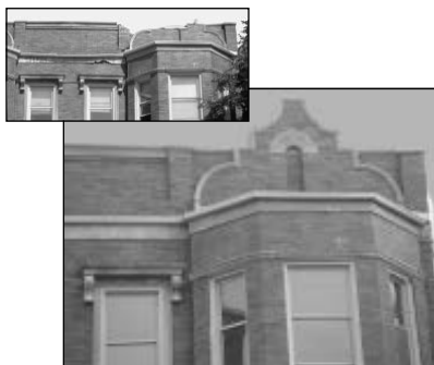
The crumbling facade on this apartment building at 4343 S. Michigan Avenue was restored to its original state through the Troubled Buildings Initiative.
