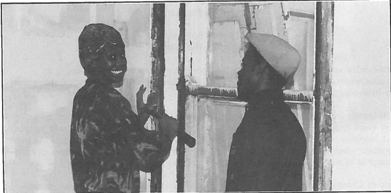
ACORN homesteaders build "sweat equity" in a southside building.
